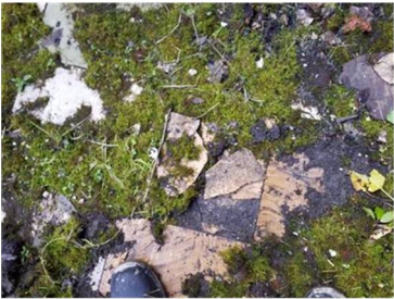
Vinyl floor tiles and bitumen adhesive
