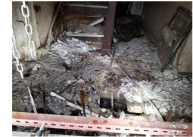
Administration Block internal
