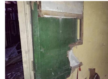
Fire Doors throughout building.
