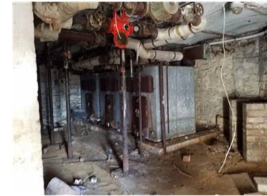
Rope seals to Boiler and Paper Gaskets
