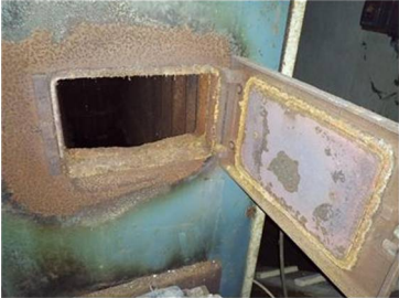
Rope Seals to Chapel Boiler
