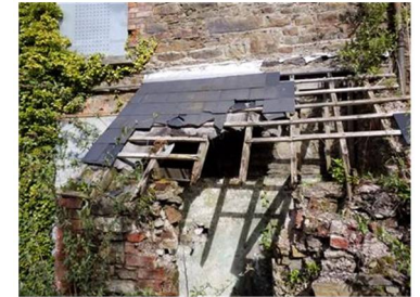
Lean too Roof slates
