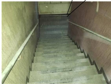
Vinyl Floor Tiles and Bitumen adhesive containing asbestos
